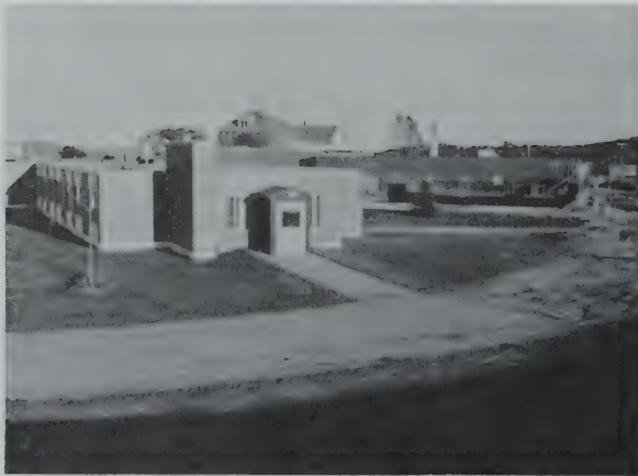
Part of Nursing Home with construction in progress.
