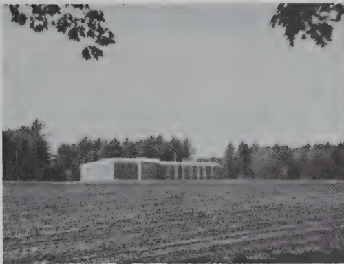
The County Administration Building which contains the Commissioners office, Business Office, Registry of Deeds, Sheriffs Dept. and Probate Court.
