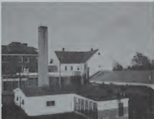
Boiler house foreground; Jail & Annex background.
