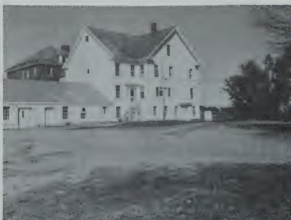
Side view of Annex Bldg. which contains Health & Home Care Services, Probation Dept., and Community Action Programs office.
