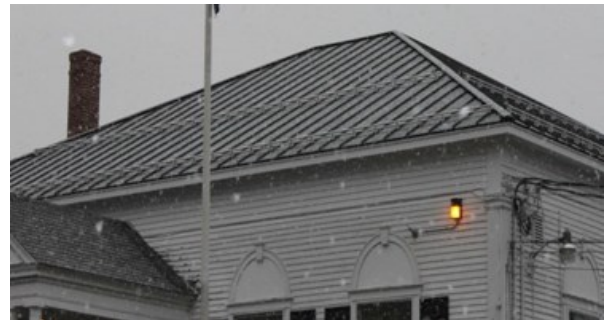
Town Hall Roof Replacement
