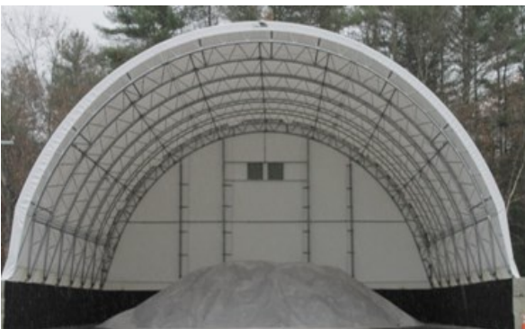
Public Works New Salt Shed
