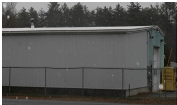
Recycling Center Roof Replacement
