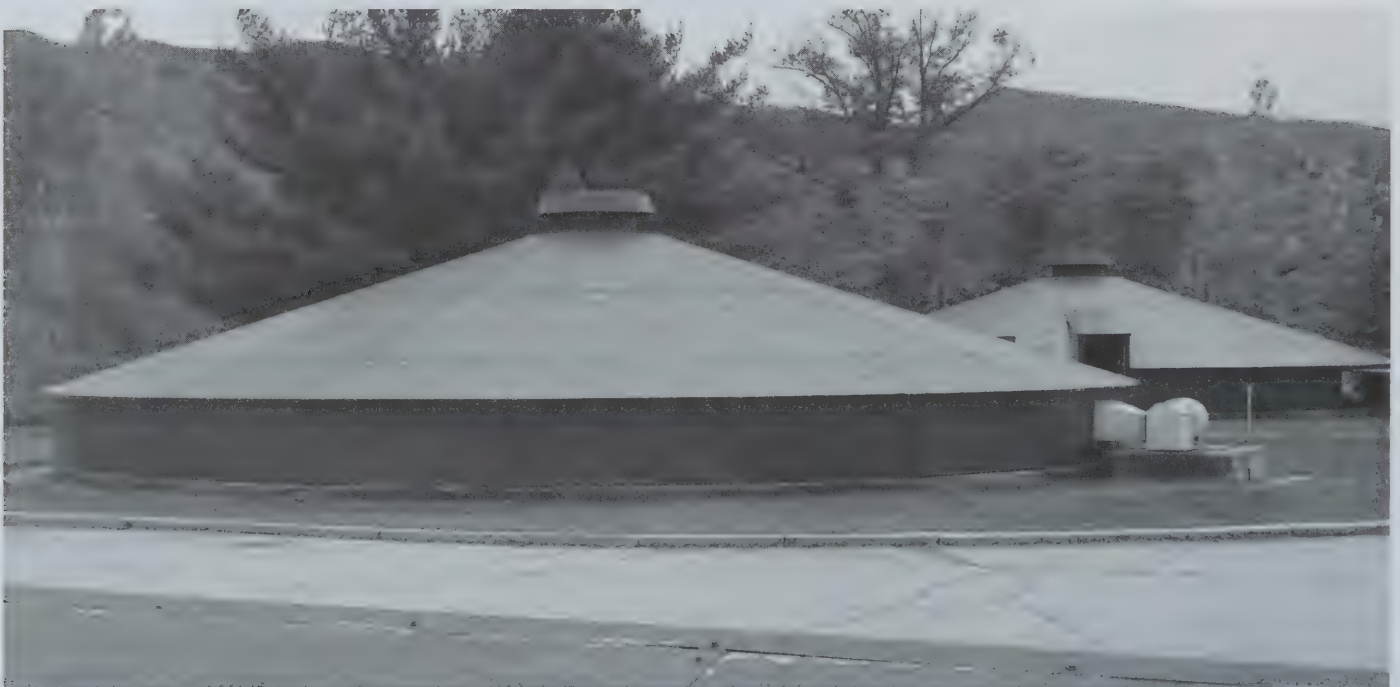
Resurfaced Clarifier Settling Tanks
