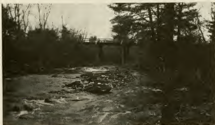
Mill Hill Bridge - c. 1900 Photo from collection of George Wentworth
