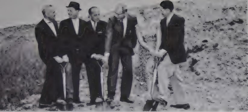
Breaking ground for first multiple dwelling at Keewaydin Shores
