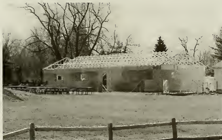
The new Tuck Building under construction.
