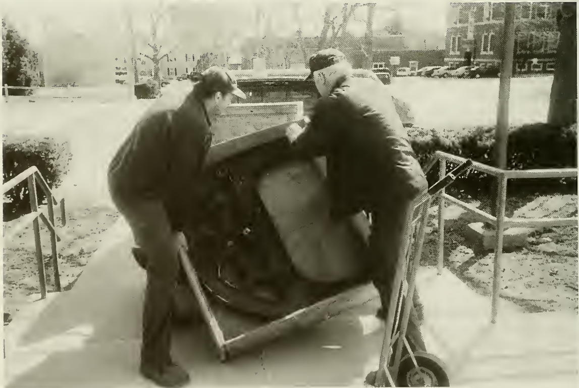
Public Works employees John O'Brien and Jim Norton carefully transport the town clock parts to the town office for safe keeping.
