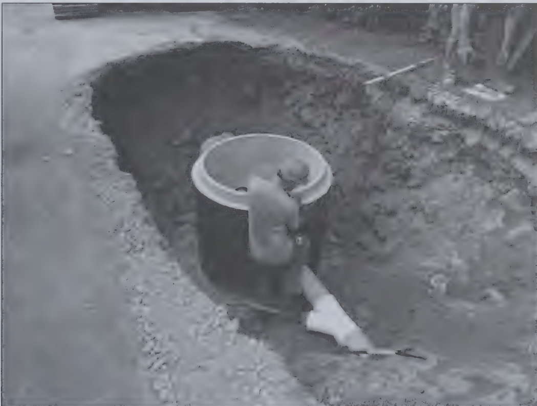
New sewer manhole installation on Willis Place
