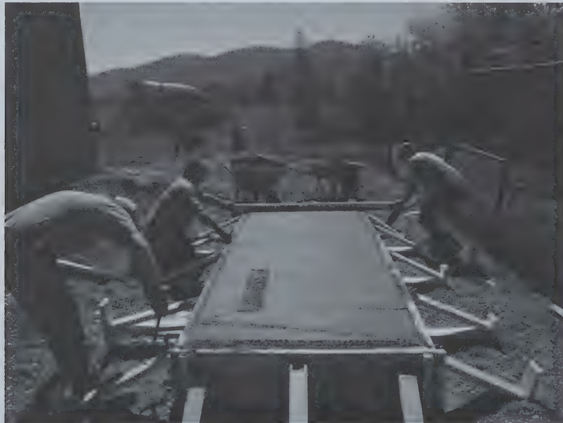
Installation of new concrete generator pad at Well # 2 by Department employees
