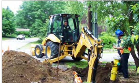
Fire hydrant installation
