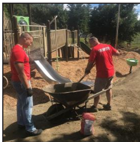
LPD Officers assisting with building the new playground at Remich Park
