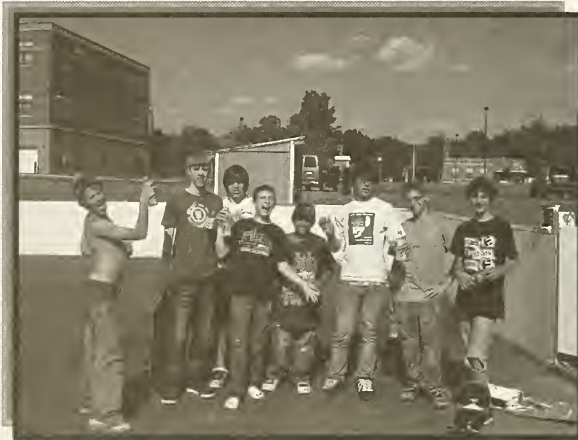
Some of the crew helping with construction of the warming hut at the Skating Rink
