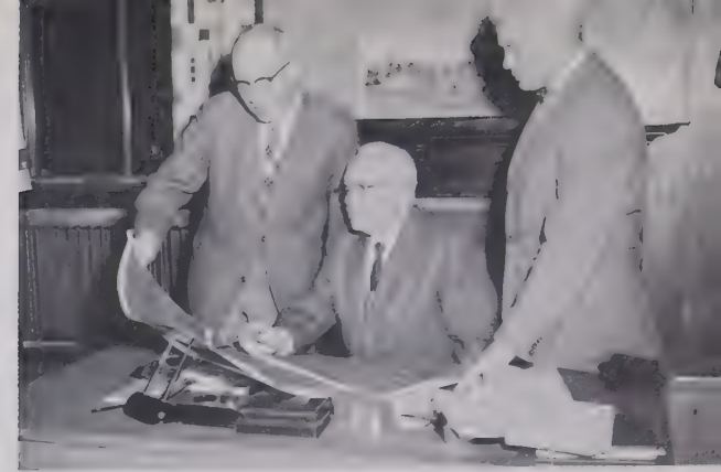
Checking plans for new school
