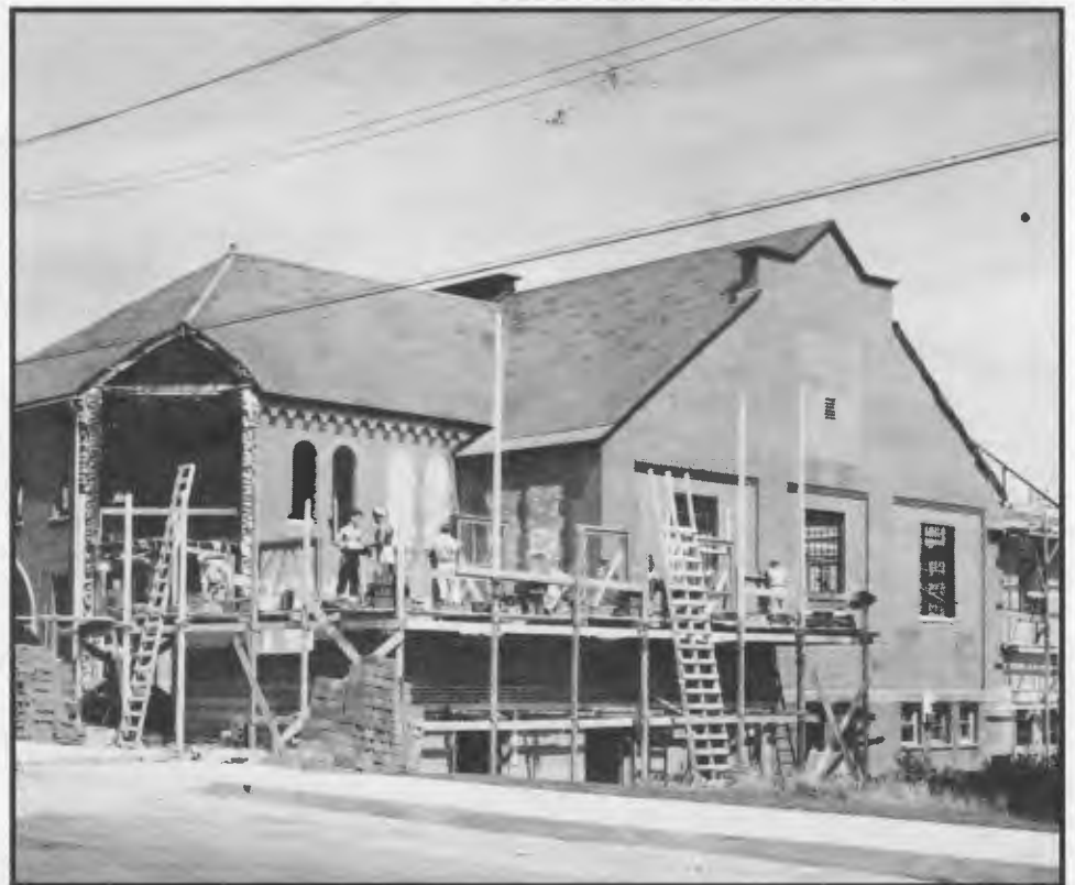
Removal of New Hampshire Hall tower 1940
