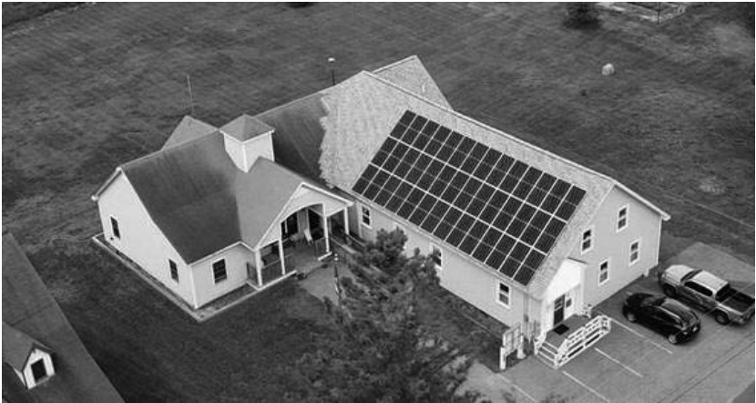
(Photo Provided by Sean Carlson of 603 Solar)
