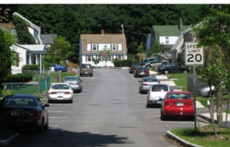
Phase I of the Raleigh Way Streetscape Project
