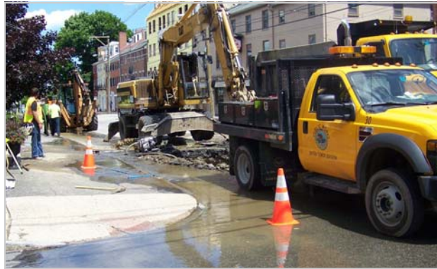
State Street Reconstruction Project
