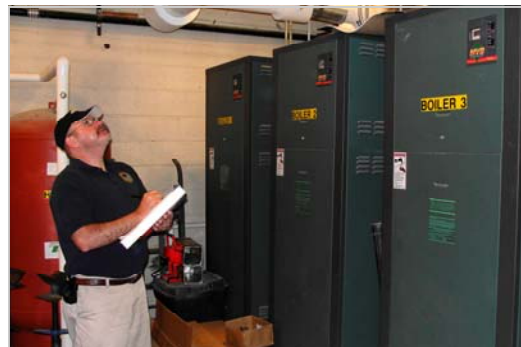
Plumbing/Mechanical Inspector Brian Kiely on the job
