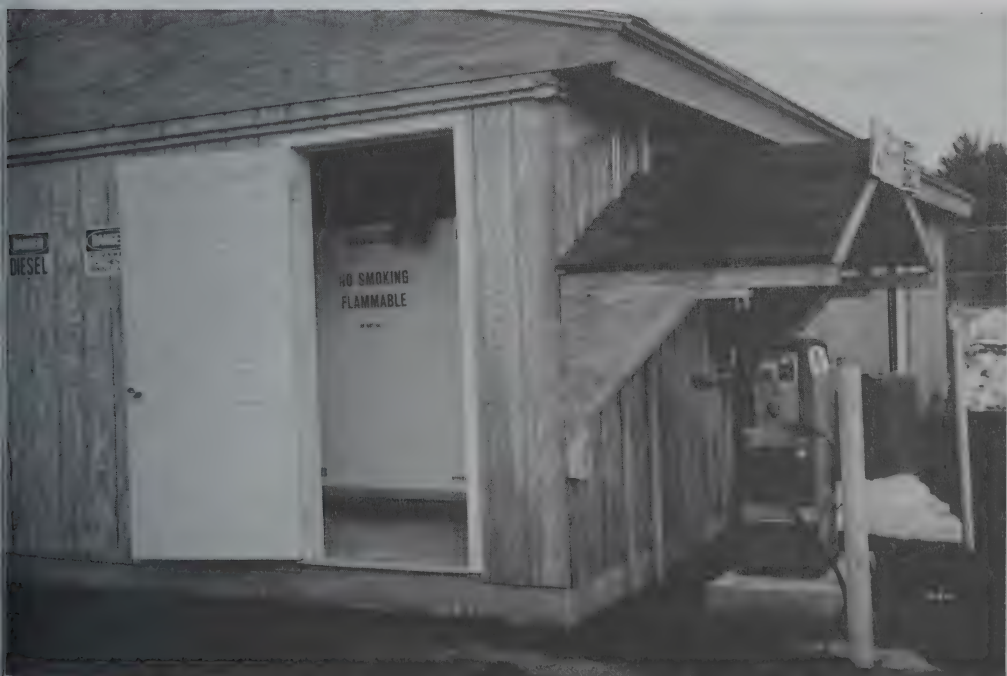
Newly constructed fuel station for town vehicles – fall of 1994 completion.
