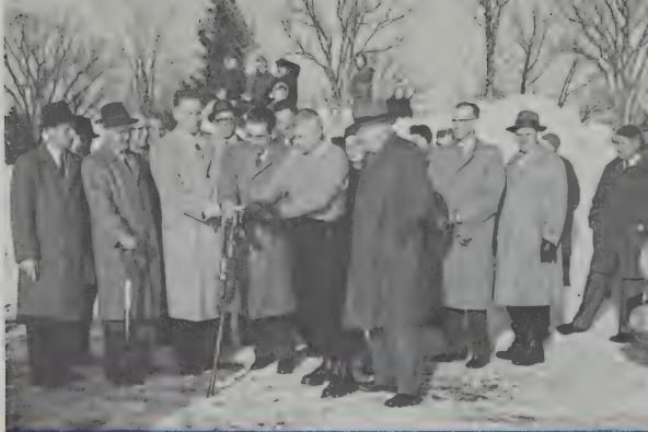
Breaking ground for new elementary school on Pleasant Street.
