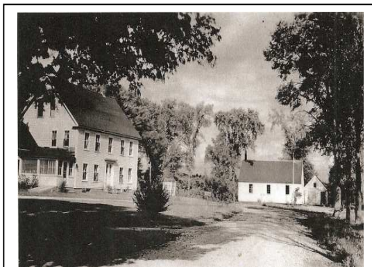
Churchill Homestead & School House
