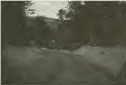
Broomstick Hill Road Construction Widening & Ditching Completed By Morrill Construction
