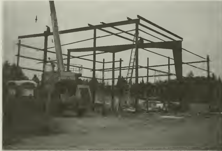
New Transfer Station Wall Framing
