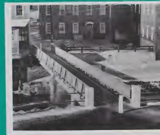
New Mill Street Bridge
