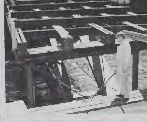
Start of Construction New Mill Street Bridge
