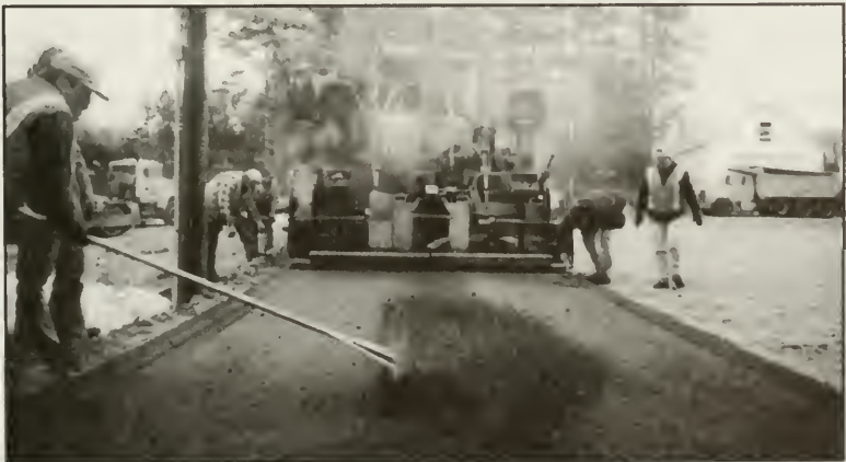
Paving of ice rink and roller blade park for recreation area
