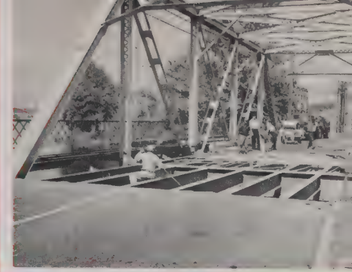
Resurfacing of Messer Street Bridge
