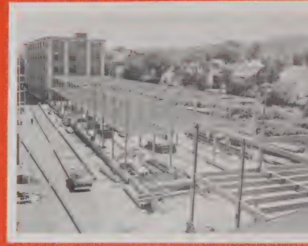
New Addition to Scott & Williams
