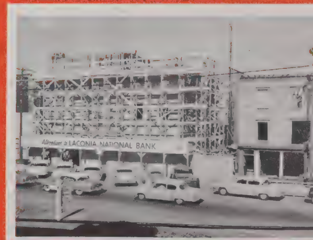
Signs of Progress on Main Street
