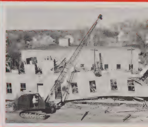
Start of New Beacon Street Parking Lot
