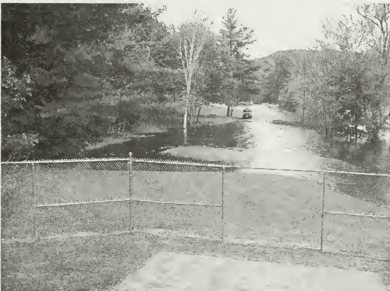
Henniker Waste Water pump station on Ramsdell Road during the flood of October 2005.
