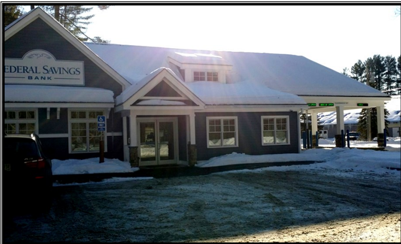
Federal Savings Bank Renovation 2017
