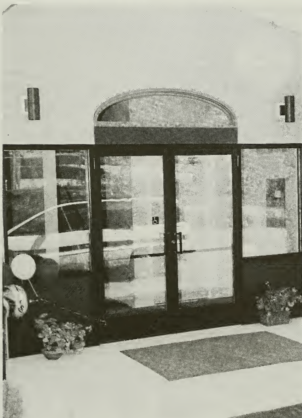
(NEW HANDICAP ENTRANCE TO THE LIBRARY)
