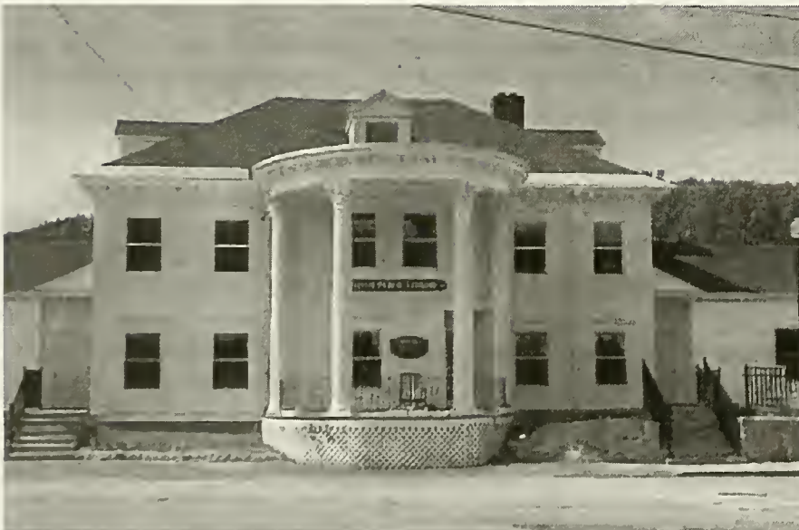
Gorham Public Library located at 35 Railroad Street
