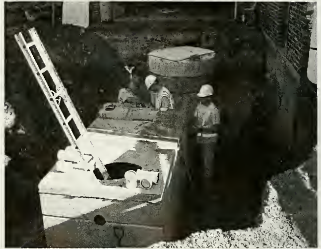
Installation of New Grease/Separator at Fire Station
