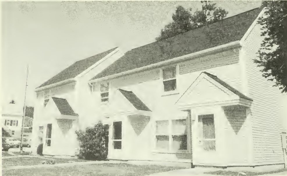
Major exterior improvements, including all new siding and guttering at Smokey Hollow Common at 225 Main Street (between Spring and Summer Streets)
