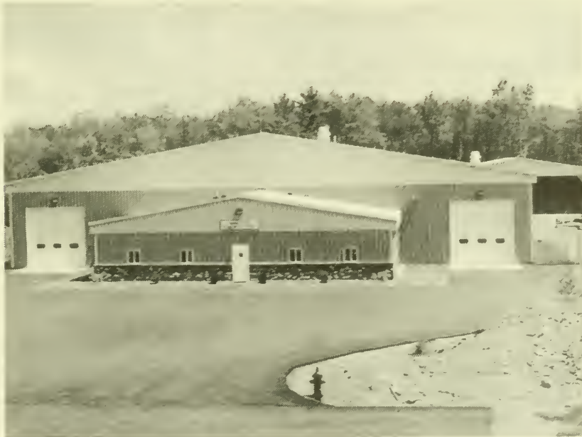
Somersworth Public Works Department
