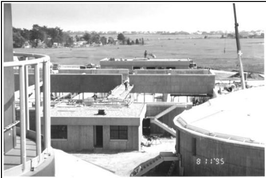
(Treatment facility during construction 08/95)
