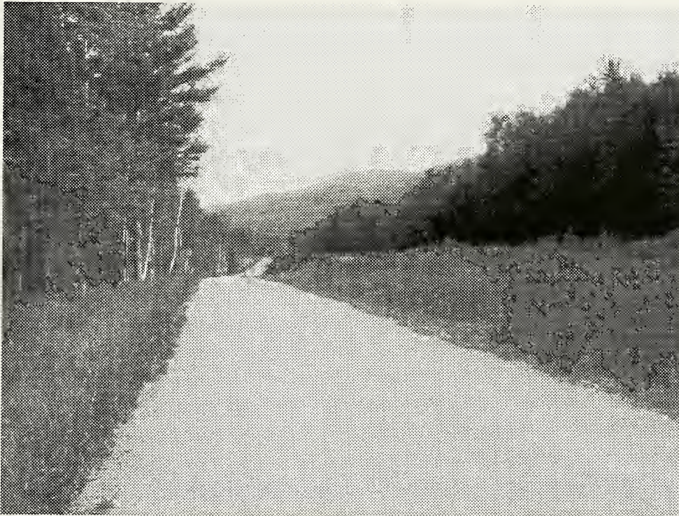
View South on the Multi Modal Path
