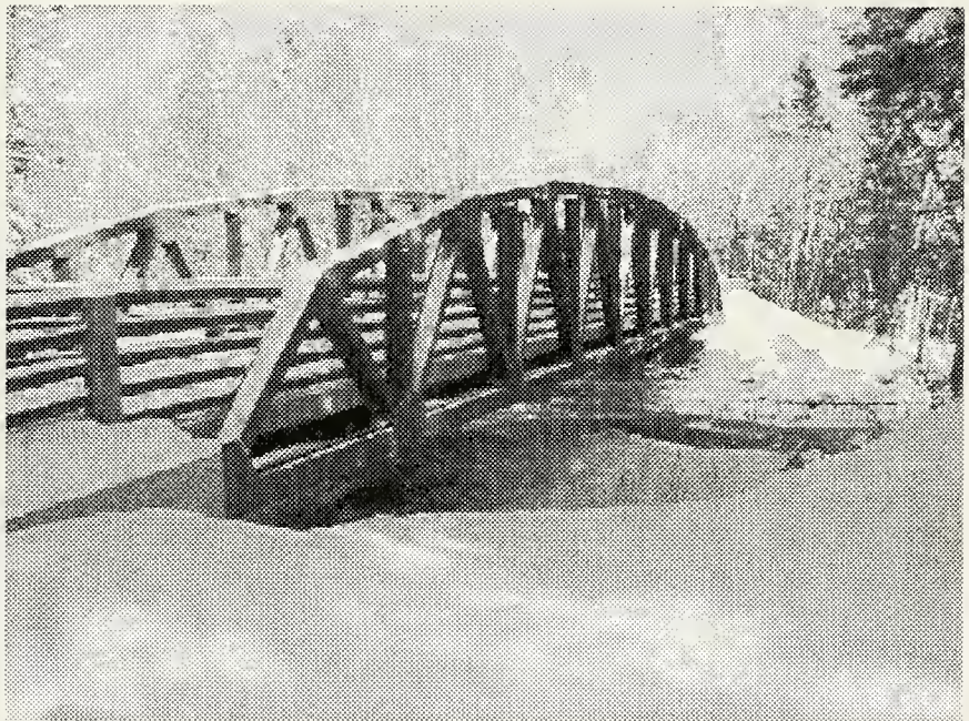
Multi Modal Path Bridge
