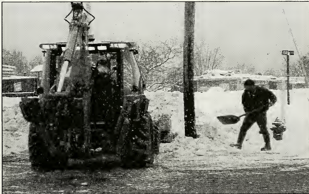
Water & Sewer Department Employees cleaning around the hydrants
