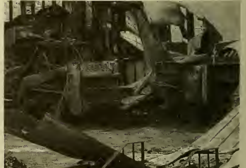
Aftermath, Transfer Station Fire
