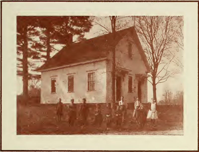
THE UPPER VILLAGE SCHOOL - BUILT 1889
