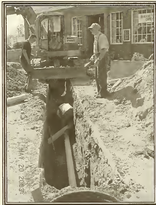
Lancaster National Bank Remodeling Project
