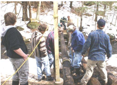
Fellow scouts and community members at work on the bridge
