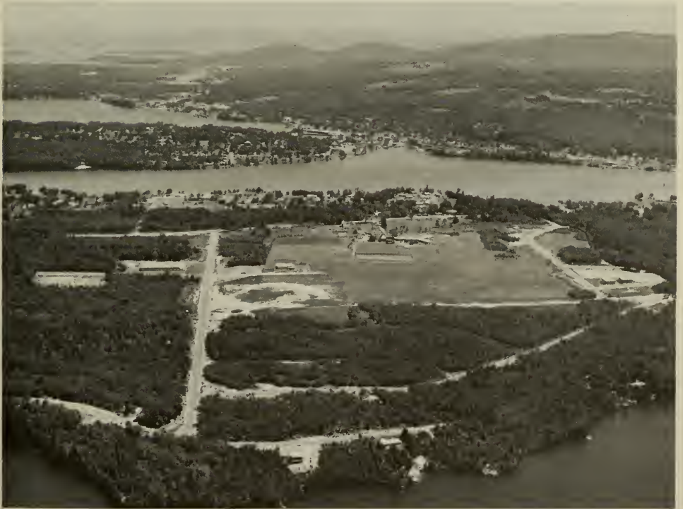
Aerial View of O'Shea Industrial Park
