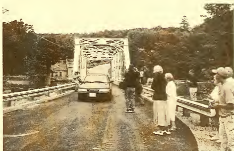
Patterson Hill Road Bridge
