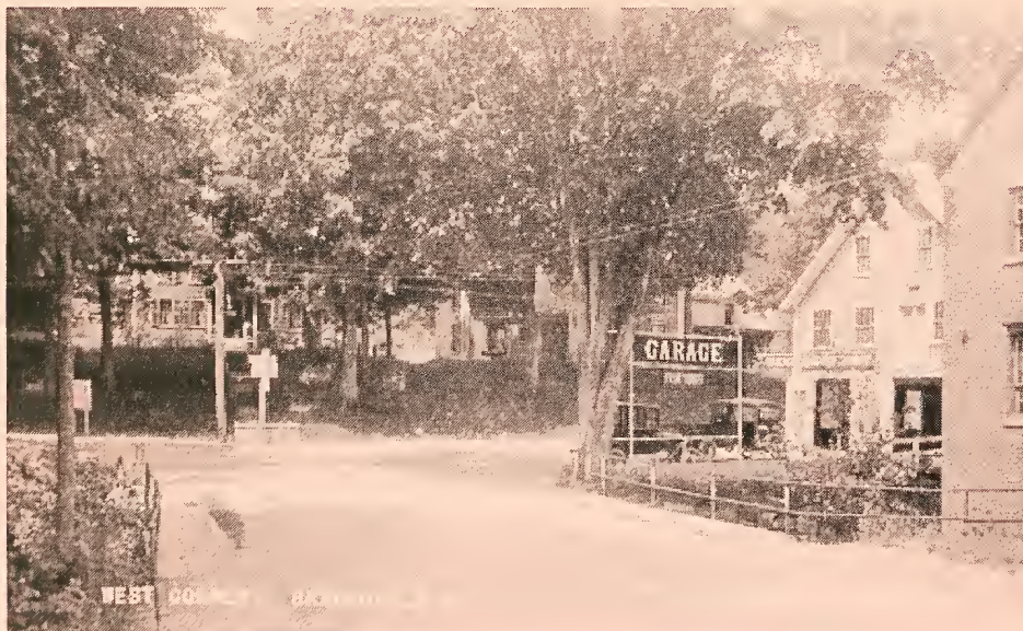
Intersection of West Main, High Street, Cochran Hill and Water Street About 1910
