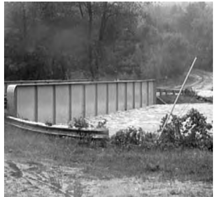
Sand Hill Bridge
