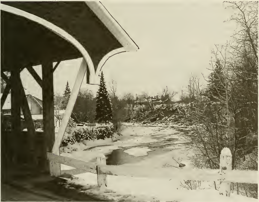
Mechanic Street Covered Bridge
