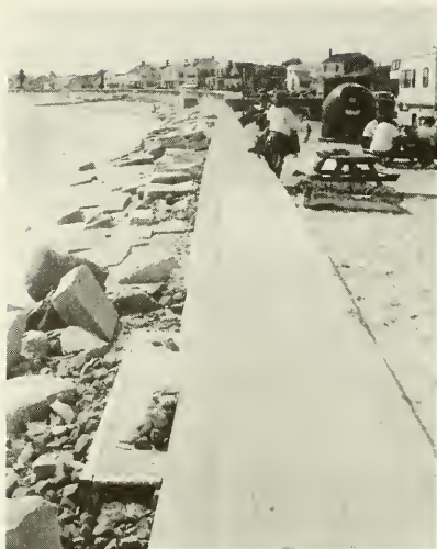
Bicentennial Park: Seawall gap filled in by DPW
