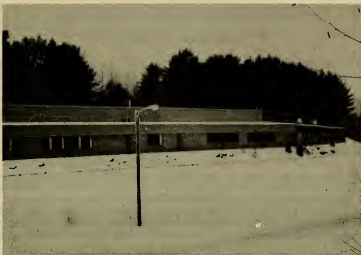
Doubling of the Tender Corporation. Added 12,000 square feet.
