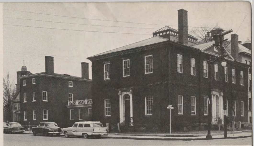
General view of Public Library showing newly renovated annex.
