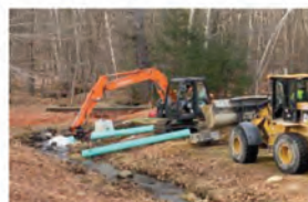
(L-R) Fox Pond drainage and inlet/outlet work and new pipe installation
