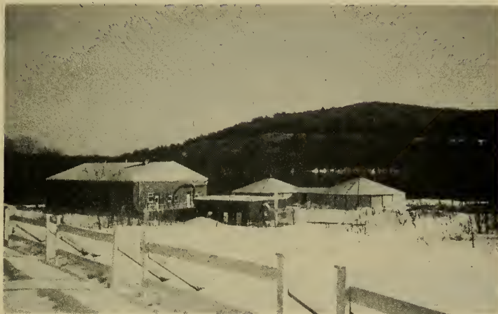
The New Secondary Wastewater Treatment Plant
