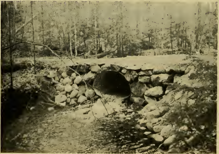
Culvert Replacement at "The Dells"
