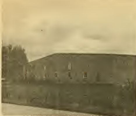
Building #1 at Industrial Park
