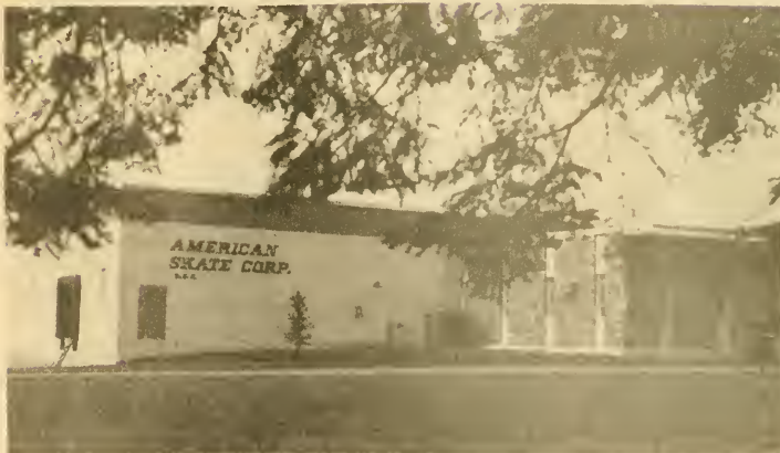
Building #3 at Industrial Park
