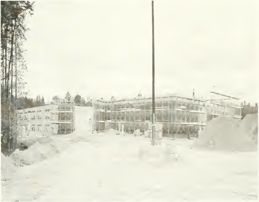
Construction of the new Middle School is Underway!
