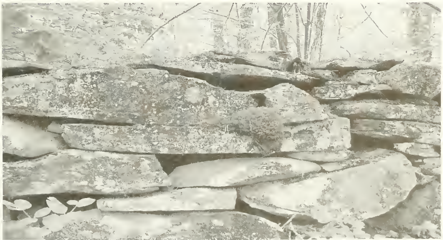
A Stone Wall on Town Farm Road
