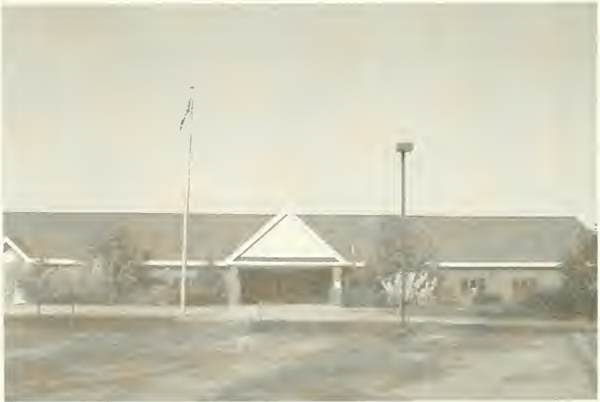
Barrington Elementary School on Route 125
