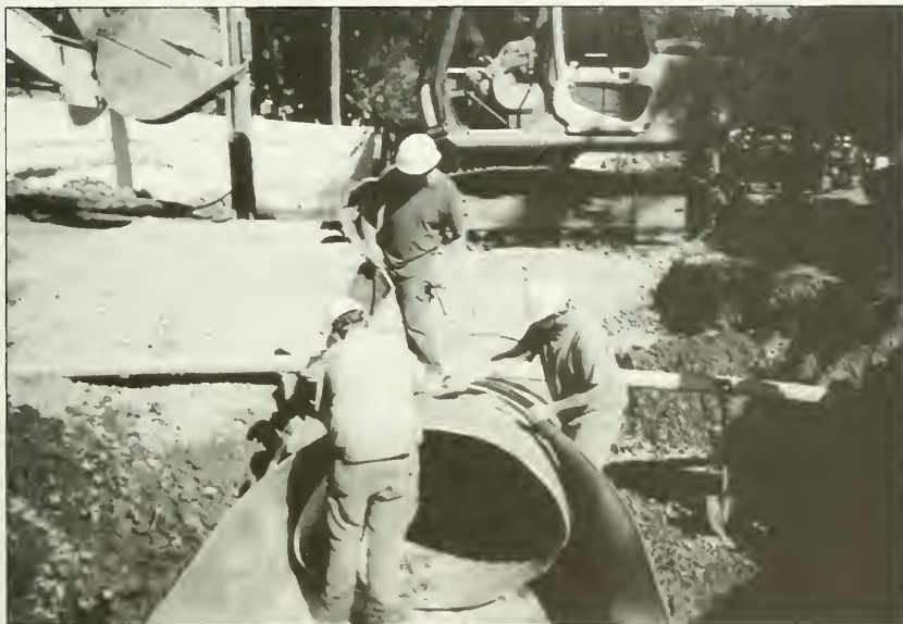
Lower Collins Street Culvert Replacement
