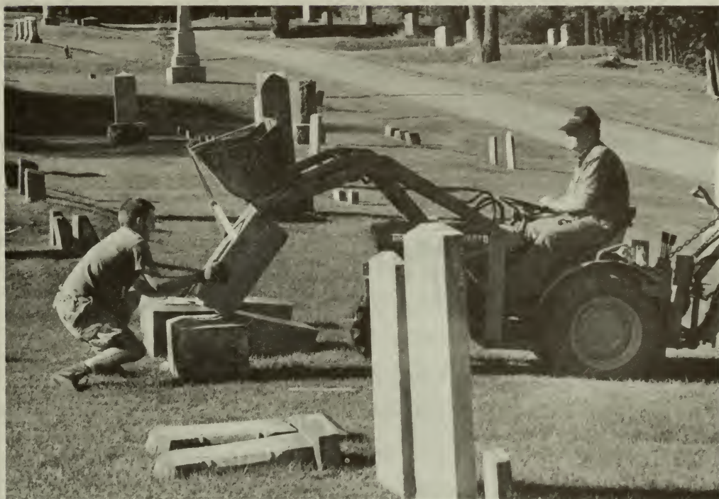
Dana Nason (on the tractor), the caretaker of Summer Street Cemetery in Lancaster, and Eric Scott working to repair headstones that had been knocked over by vandals.
