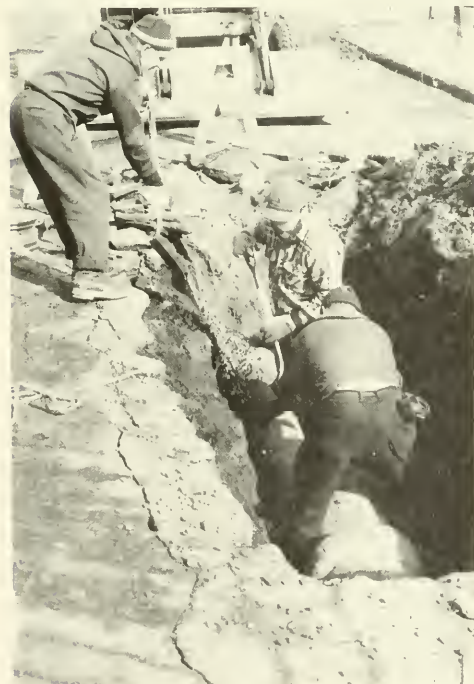
Public Works crew repairing surface water drain on Denmark Street
