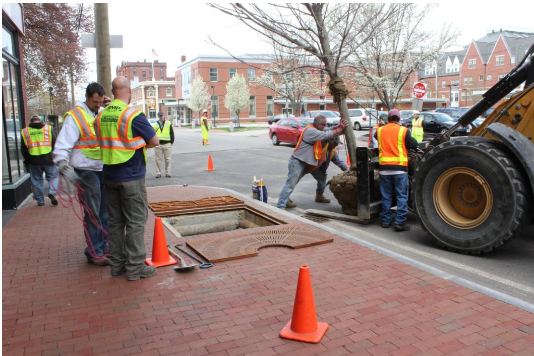
Photo 16: The red maple is being delivered to tree box filter site.
