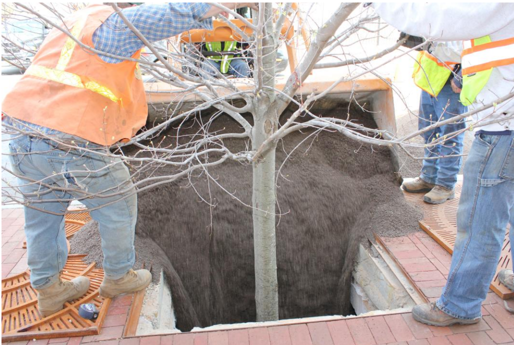
Photo 18: Soil mix is being added to box.
