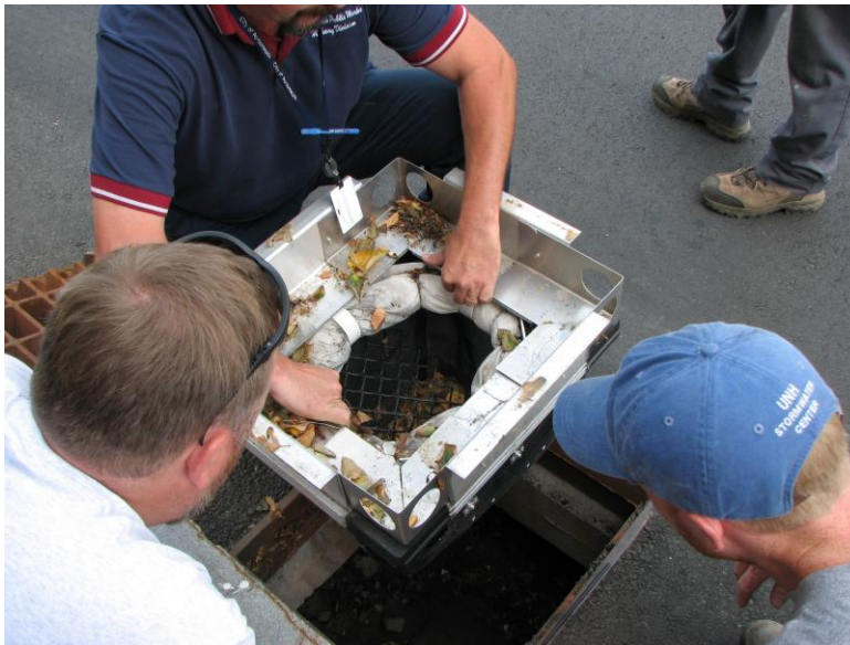
Photo 6: Drop inlet debris catcher is installed in catch basin.
