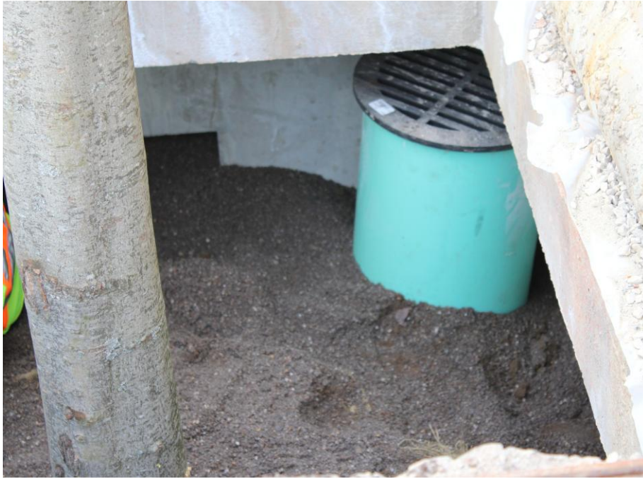
Photo 2: A high flow bypass pipe helps divert water from the box into the stormwater system when stormwater volumes are especially high.
