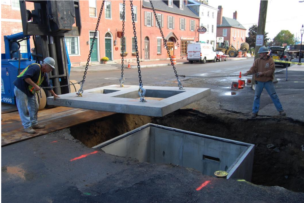
Photo 11: The cover is placed on the box.
