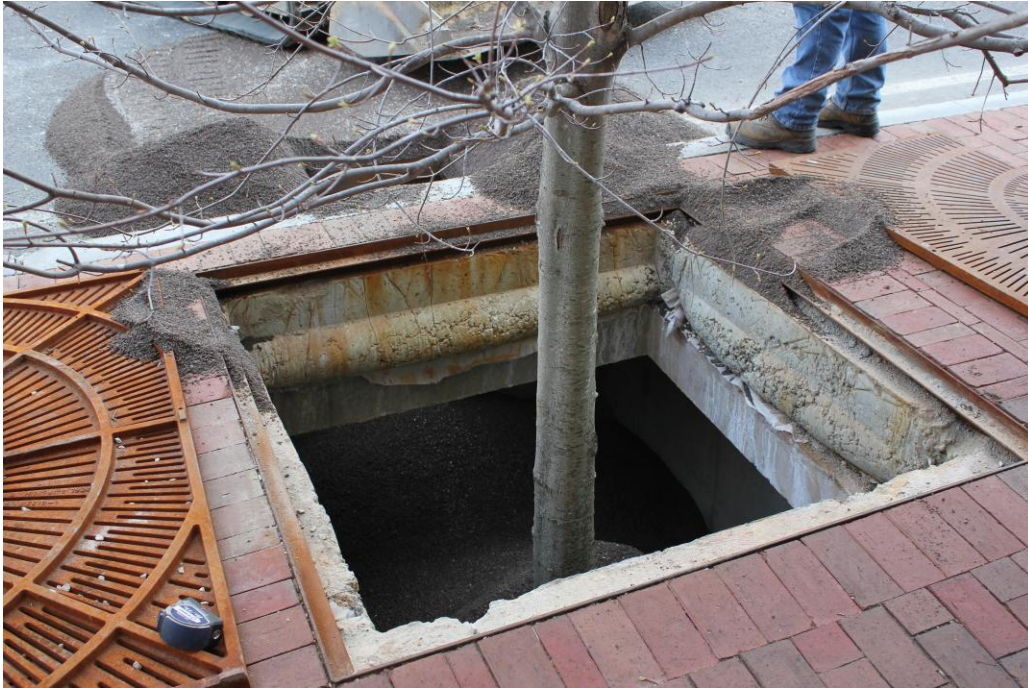
Photo 17: Note depth of planting required to fit this box and installation.
