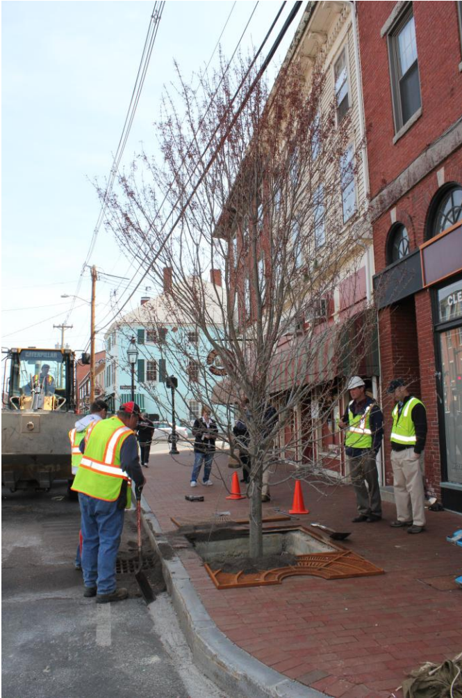
Photo 19: The tree box filter undergoes a final inspection.
