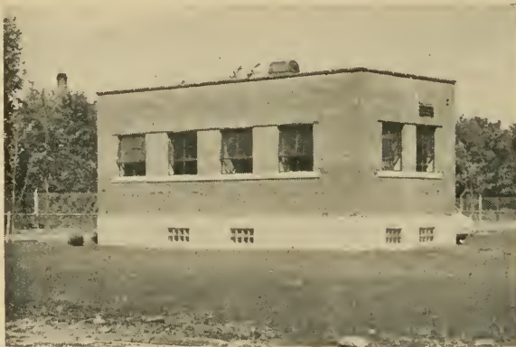
A. The Rack House
