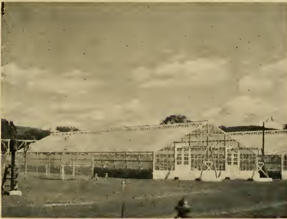
E. The Sludge Drying Beds
