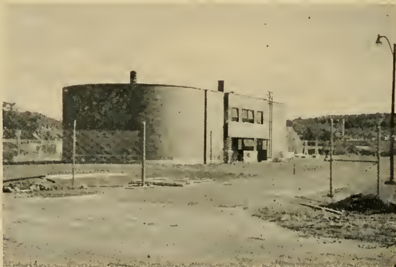
D. The Sludge Digester
