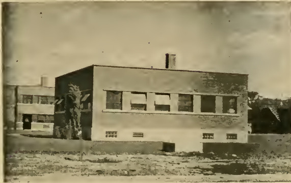
B. The Pumping Station
