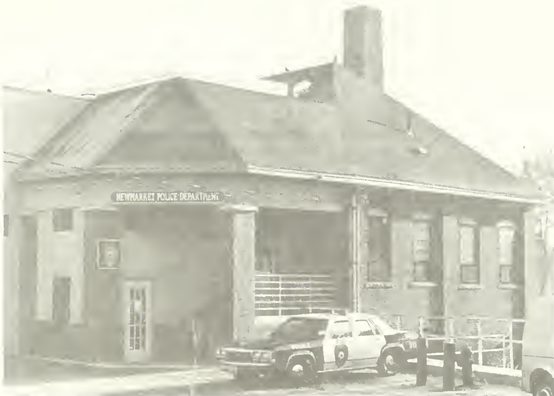
NEWMARKET POLICE DEPARTMENT AND WATER TREATMENT PLANT
